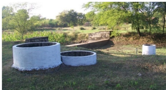
Figure-4 Check dam with recharge pit for recharge of rainwater in Nagpur central India
